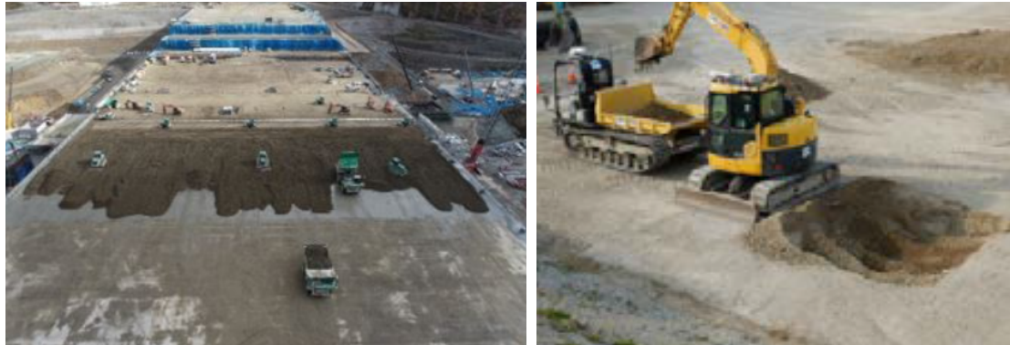
(a) Work in dam construction [8]
