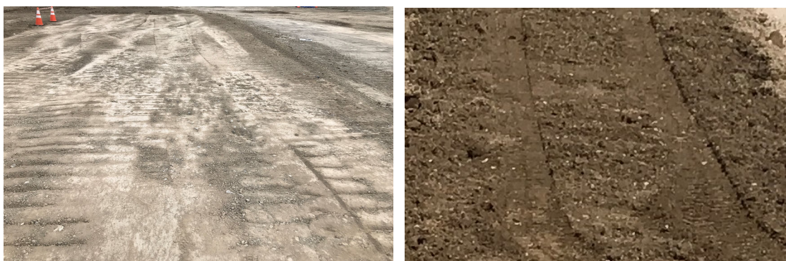
(a) Hard (roller compacted) ground surface (b) Soft (uncompacted) ground surface
